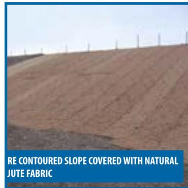
RE CONTOURED SLOPE COVERED WITH NATURAL JUTE FABRIC
